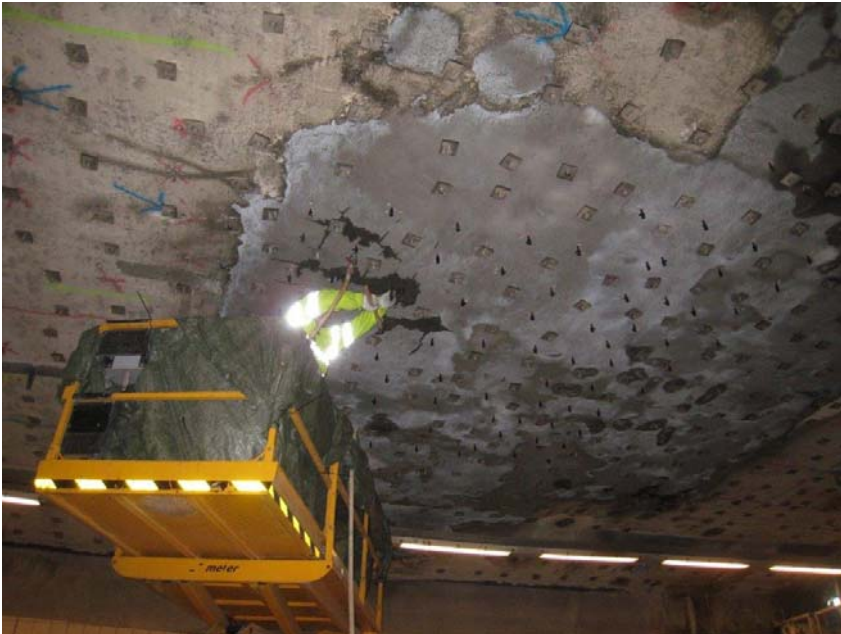
Figure 4.5-4 Injection of leaking cracks
