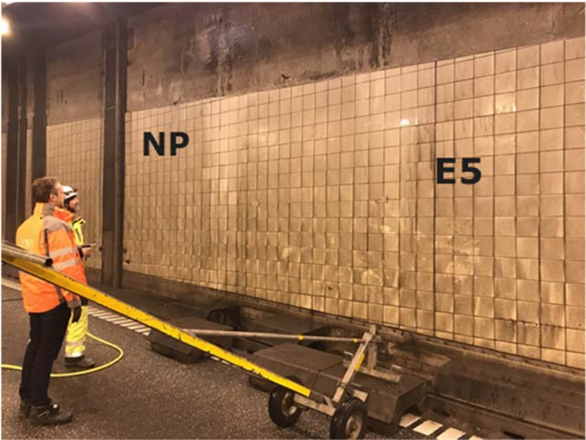
Figure 6.7-1 Closure joint between Northern Portal (NP) and Element V (E5) before removing tiles and concrete in order to inspect the reinforcement.
