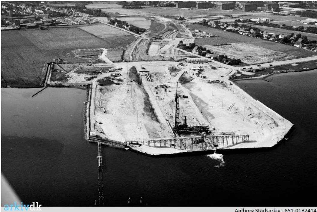
Figure 4.3-1 Dry pit at northern shore for casting of in-situ tunnel, portal building and ramp.
